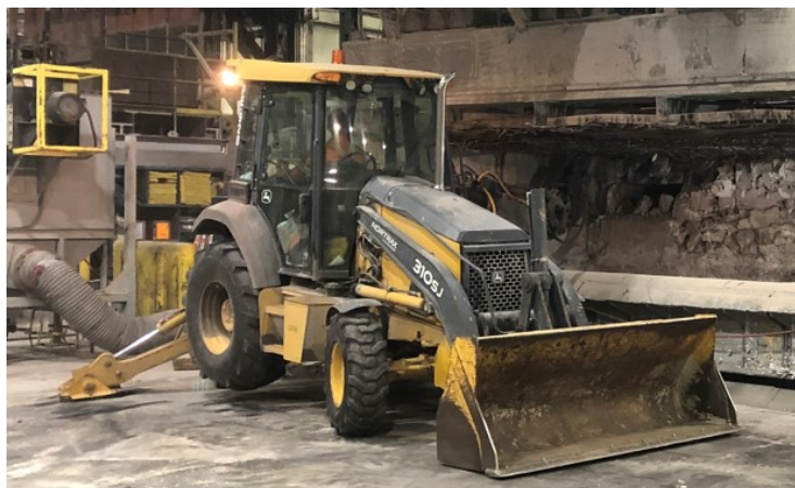
Figure 2. Typical backhoe used for furnace demolition (author's image).
